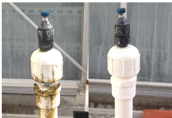
Figure 2. The mist nozzle on the left is a source of algae during propagation, while the mist nozzle on the right is properly cleaned.
