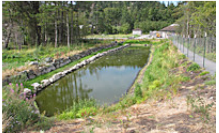
Figure 2. Constructed wetlands can be effective at removing some agrichemicals. Photo: Courtesy of Cleanwater3.org.
