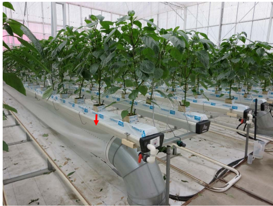
Figure 1. Example of a closed-loop irrigation system. The channels under the rockwool slabs collect the nutrient solutions that runoffs from the substrate (note red arrow). The solution is then treated and stored until it is pumped back into the crop.
