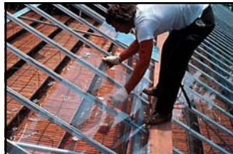
Laying panes on sash bars
