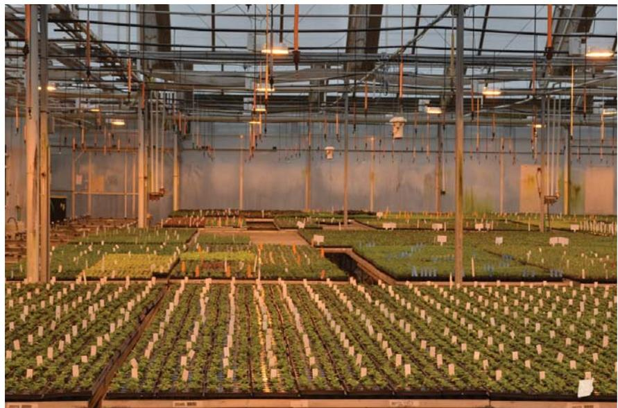
Figure 1. Midwest greenhouse using supplemental lighting from high-pressure sodiums lamps to provide  $70 \mu\text{mol}\cdot\text{m}^{-2}\cdot\text{s}^{-1}$  to their young plants.
