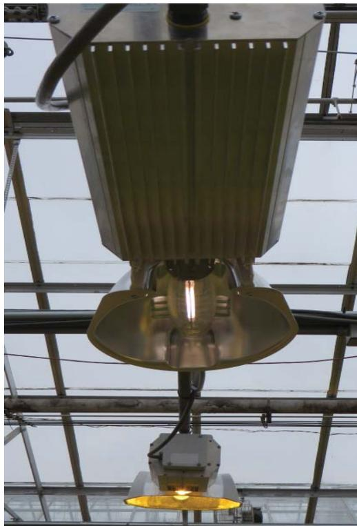
Figure 6. Dim HPS lamps that should be replaced.
