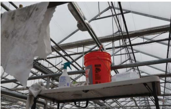
Figure 4 (right) Reflector and lamps with dust and water spots.
