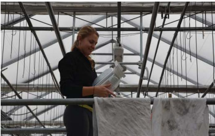
Figure 3 (left). High-pressure sodium lamp reflector has been removed from the fixture and is ready to be cleaned. Note how dirty the cloth is after cleaning just a few reflectors.
