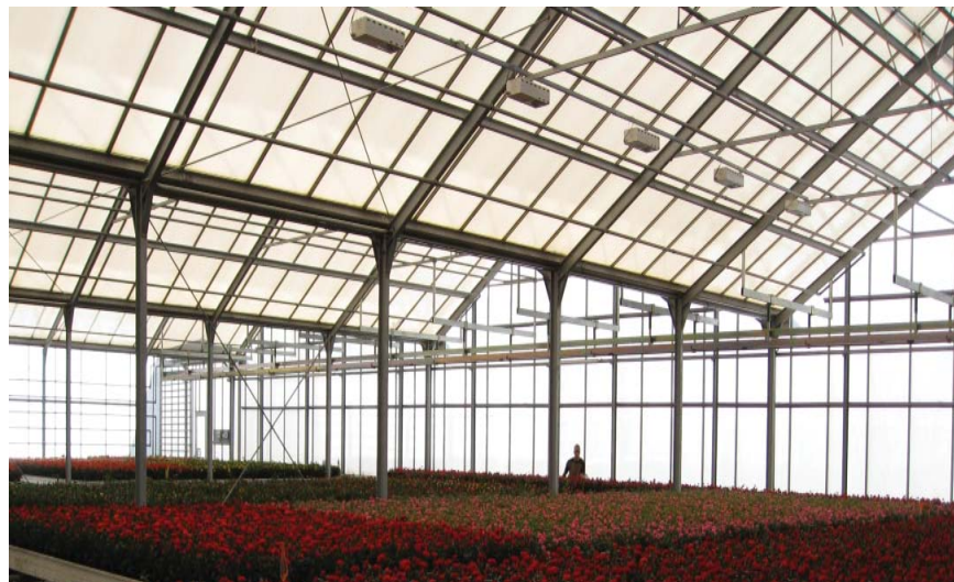
Figure 2. Glass-glazed greenhouse with whitewash on the exterior.
