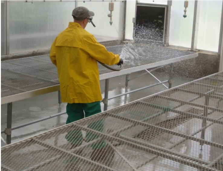
Figure 5. Greenhouse interior being cleaned with pressurized water after all plants have been taken out. Photo credits: https://pestadvisories.usu.edu/2020/01/17/greenhouse-sanitation/
