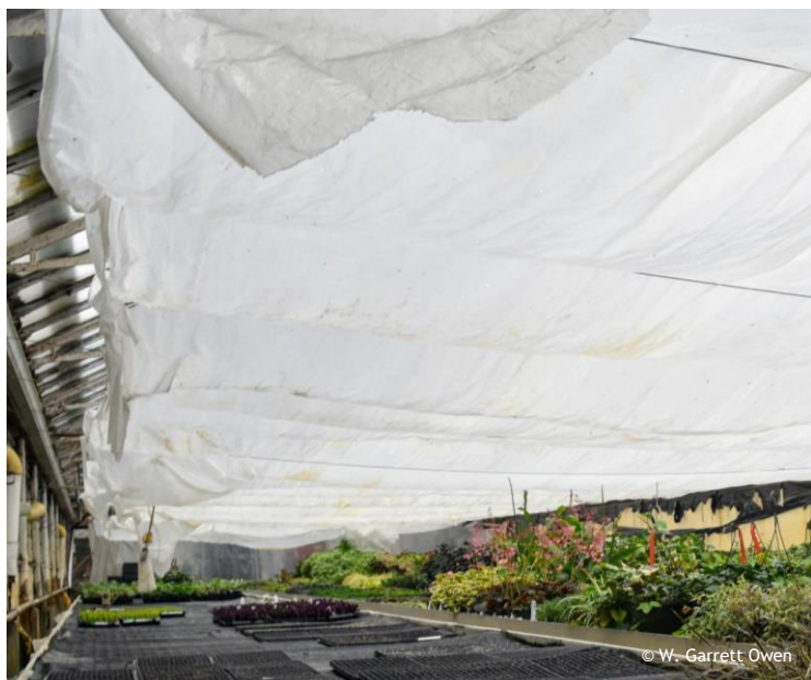
Figure 9. Example of temporary plastic sheeting used to create a barrier in a propagation greenhouse. The barrier keeps the heat air closer to the crops and prevents loss and cold air from contacting plant material. Photo by: W. Garrett Owen, OSU.
