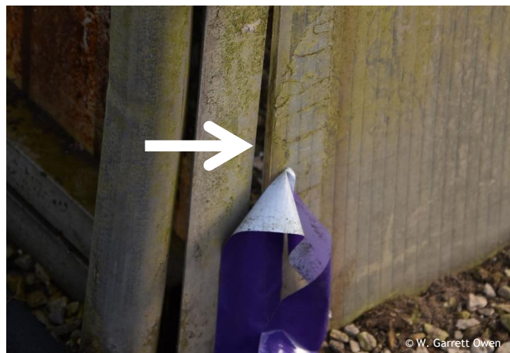
Figure 3. Example of a gap where the greenhouse end wall and sidewall meet. The gap allows cold air to infiltrate into the greenhouse environment. The gap was temporarily repaired with blue tape to prevent cold air infiltration. Photo by: W. Garrett Owen, OSU.
