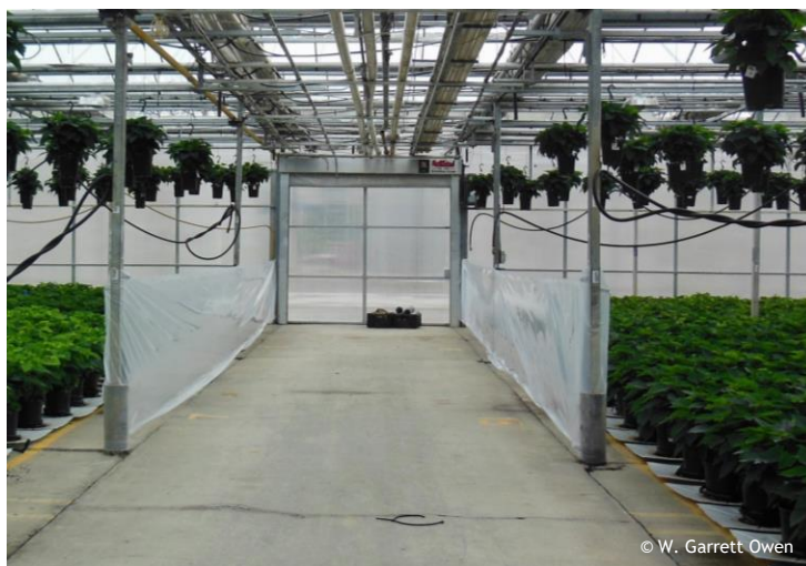
Figure 7. Example of plastic strip curtains installed near a high-traffic door to reduce the volume of cold air reaching a poinsettia crop when the doors are opened. Photo by: W. Garrett Owen, OSU.
