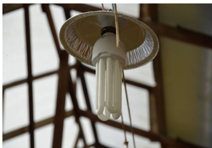
Fig. 5. A screw-in compact fluorescent lamp (CFL) with a reflector pie plate used in greenhouses to provide LDs.
