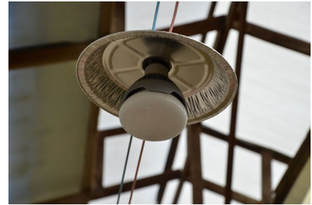
Fig. 3. A screw-in LED photoperiod lamp (currently available in Europe) with a pie plate reflector.
