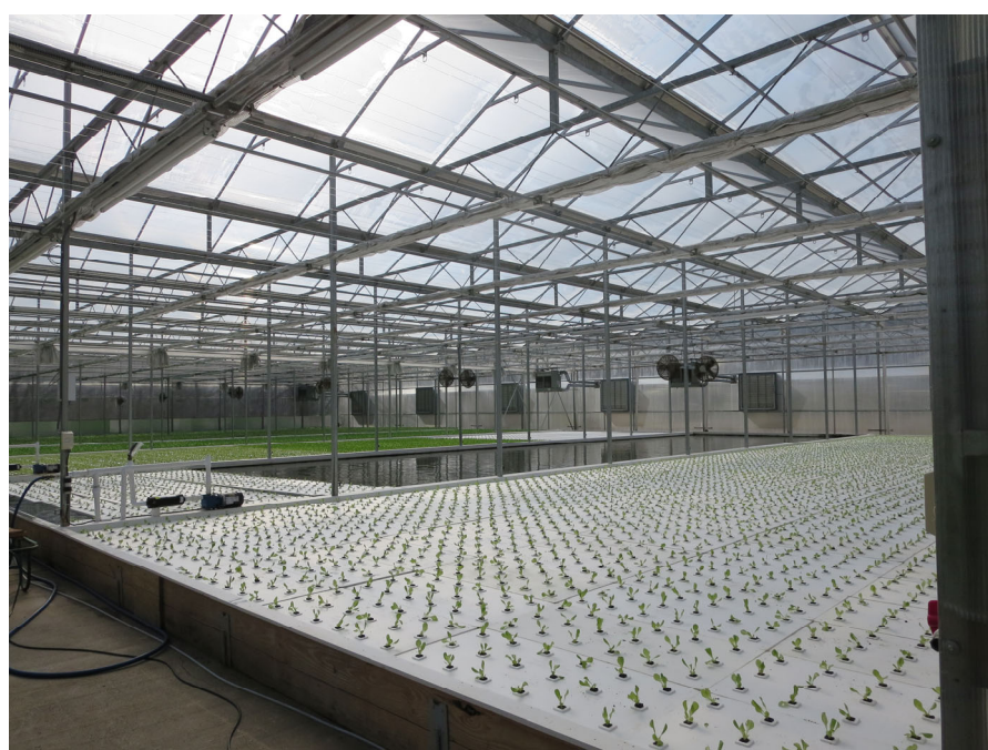
Figure 1. Materials observed in a typical greenhouse producing hydroponic crops in deep water culture include metal columns, polystyrene foam (Styrofoam) boards, concrete floors, plastic liner, wood production tanks, and polycarbonate or glass walls.
