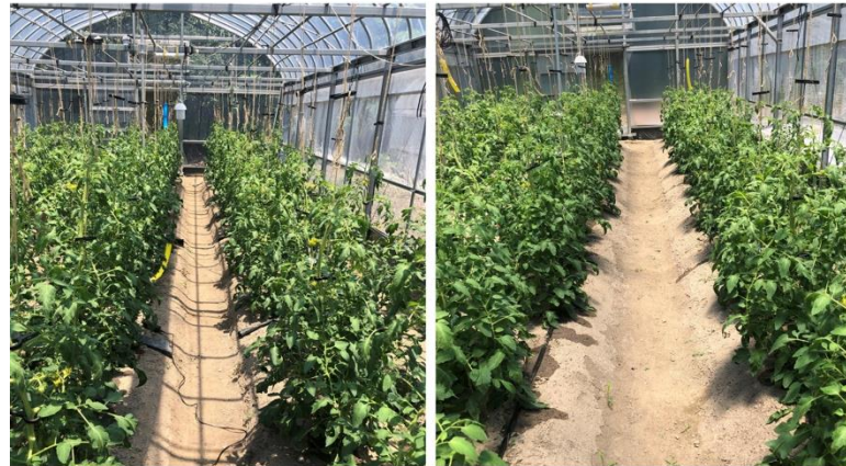
Figure 2. Greenhouse covered with a diffuse film does not create distinct shadow patterns on the floor (right). In contrast, a reference greenhouse covered with a clear film shows shadows by greenhouse structural components. Both photos were taken on the same clear sunny day (photo credit by AGC Green-Tech Co., Ltd.)
