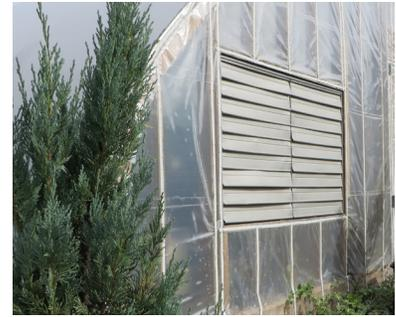
Photo 2. Repair or replace louvers so that they close tightly.
