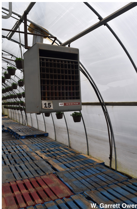
Figure 3. Primary heater used to heat the growing environment.
