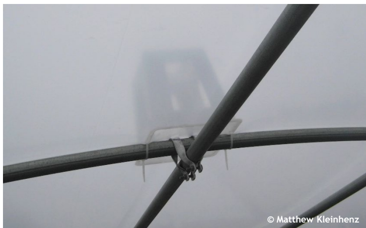
Figure 11. Greenhouse spacer blocks are an alternative to inflation blowers, offering a passive solution that doesn't require electricity, especially if electricity is limited or not available. Photo by: Matthew Kleinhenz, OSU.
