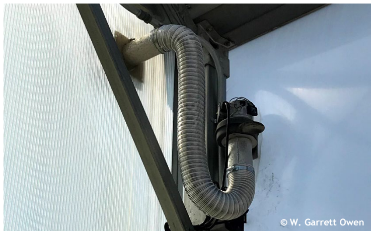
Figure 5. An example of an inflation blower using outdoor air rather than greenhouse air to inflate the two layers of double-poly. Photo by: W. Garrett Owen, OSU.
