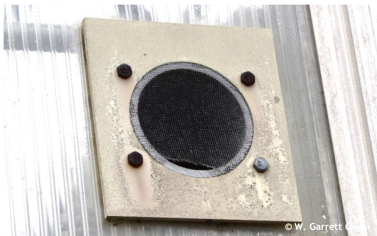
Figure 9. Example of an inflation blower fan intake that was covered with fine-wire mesh to prevent large insects and birds from nesting and obstructing air flow. Photo by: W. Garrett Owen, OSU.
