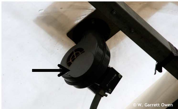
Figure 4. Example of an inflation blower manufactured with a damper that is used to control airflow and prevent overinflation and damage the glazing material. Photo by: W. Garrett Owen, OSU.
