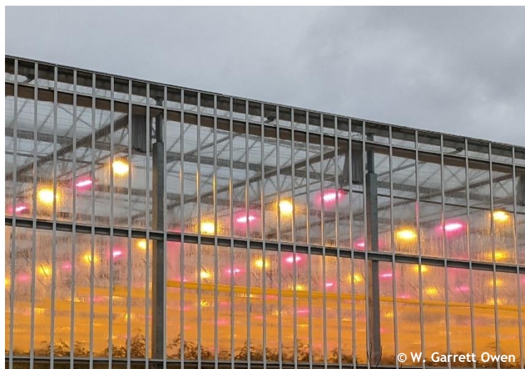
Figure 13. Example of hybrid supplemental lighting from high-pressure sodium lamps and light-emitting diode arrays deployed to increase daily light integral. Photo by: W. Garrett Owen, OSU.
