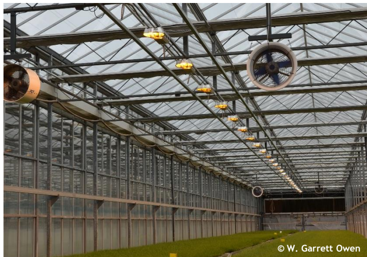
Figure 12. Example of supplemental lighting from high-pressure sodium lamps to increase daily light integral. Photo by: W. Garrett Owen, OSU.
