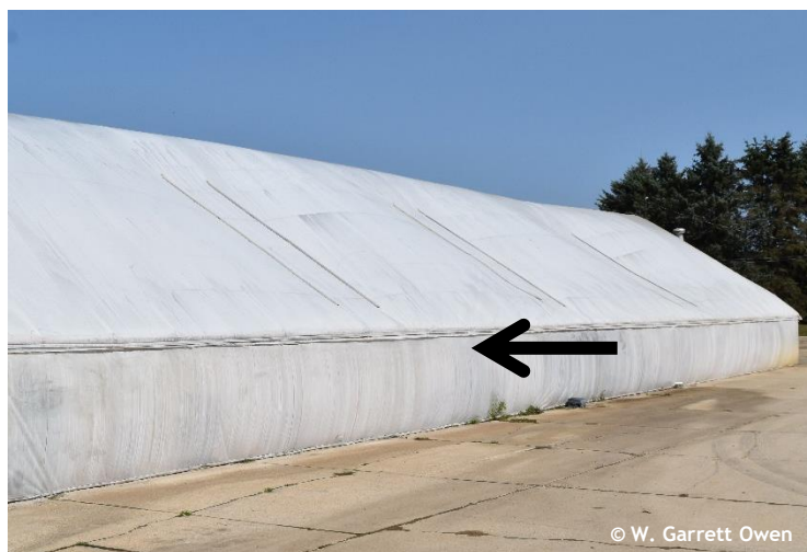
Figure 16. Seasonal application of greenhouse whitewash utilized to limit solar ambient light into the greenhouse environment, thereby reducing daily light integral. Photo by: W. Garrett Owen, OSU.
