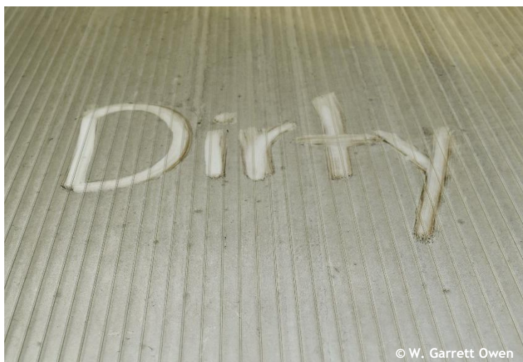
Figure 14. Dirty twinwall polycarbonate limits ambient solar light into the greenhouse environment thereby reducing daily light integral and negatively influencing transplant growth and development. Photo by: W. Garrett Owen, OSU.
