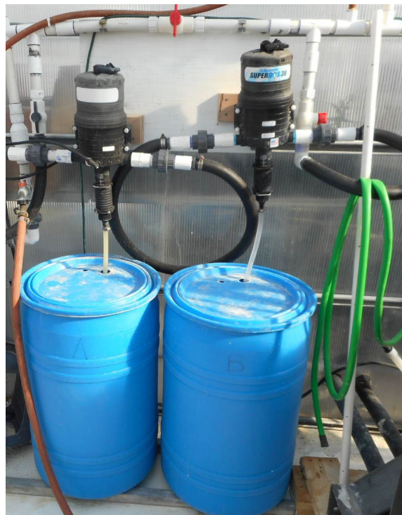
Figure 1. Two fertilizer injectors, each with a concentrated stock tank, connected in series to dispense a 2-part fertilizer. Photo: N. Mattson, Cornell University.
